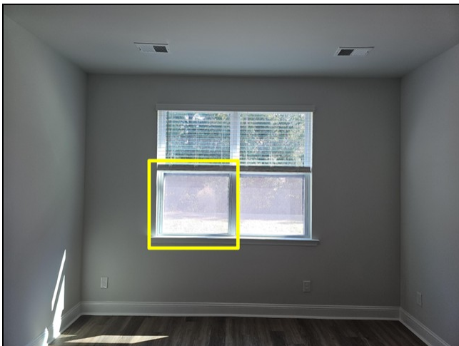
primary bedroom: difficult window
