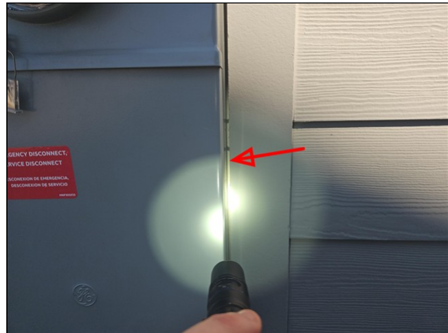
weather-resistant barrier visible
