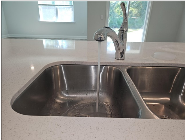
water had sulfur odor
