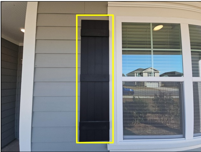
exterior walls were not painted behind decorative shutters
