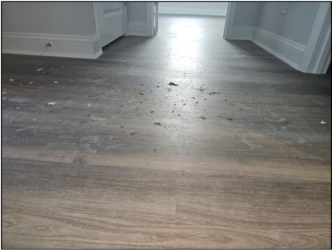
construction debris strewn on interior floors
