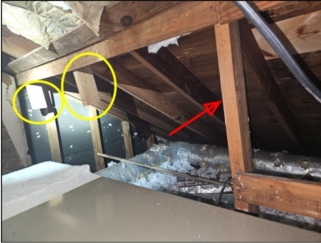
roof knee-wall bracing was modified in attic
