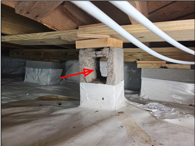
open cores should be vertically oriented
