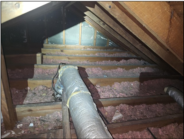
compacted blown-in fiberglass insulation in the attic
